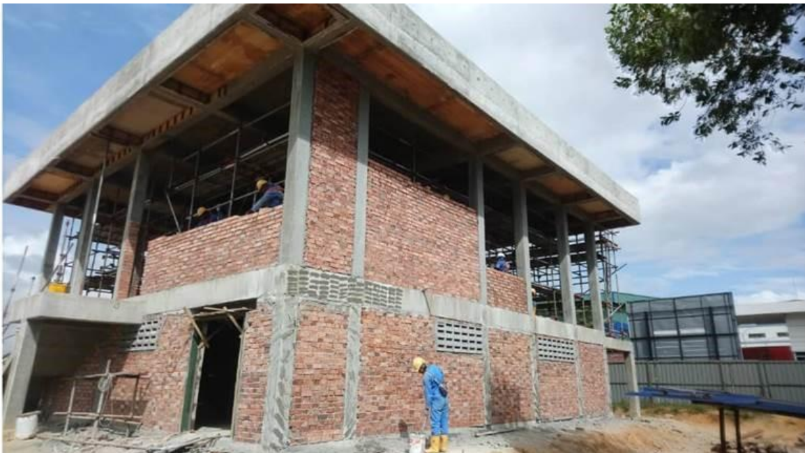
Figure 1 – Electrical substation construction
